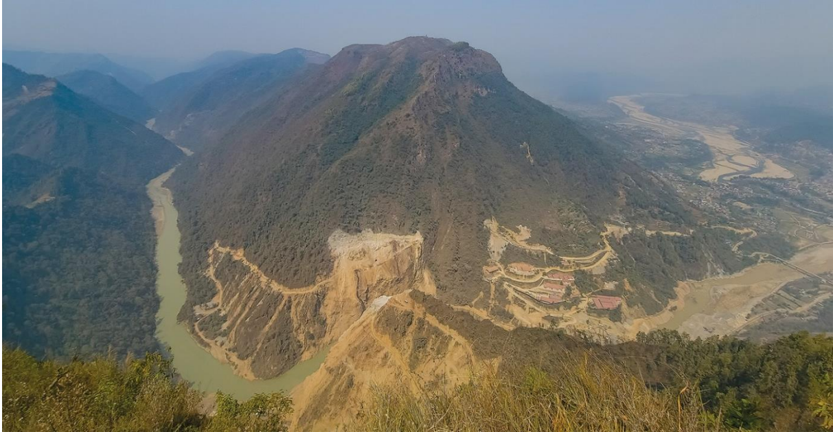
GREEN ENERGY: Dam site of the under-construction Tanahu Hydropower Project with a 25km long reservoir which will be completed in May 2026. The concrete dam will be 140m in height and hold 295 million m 3 of monsoon runoff (Tanahu Hydropower Ltd.)
